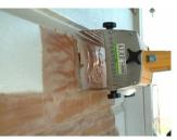
The Speedheater in action removing paint from weatherboards.
